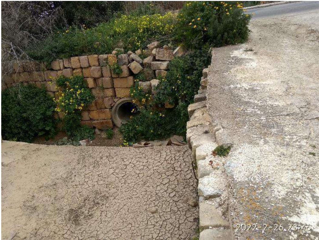
FIGURE 64: PIPELINE UNDER THE ROAD
