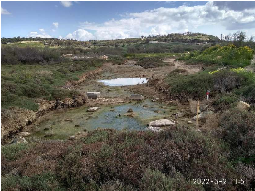
FIGURE 59: ALMOST COMPLETE DESICCATION OF POOL NO. 3 AS NOTED ON 2 ND MARCH, 2022
