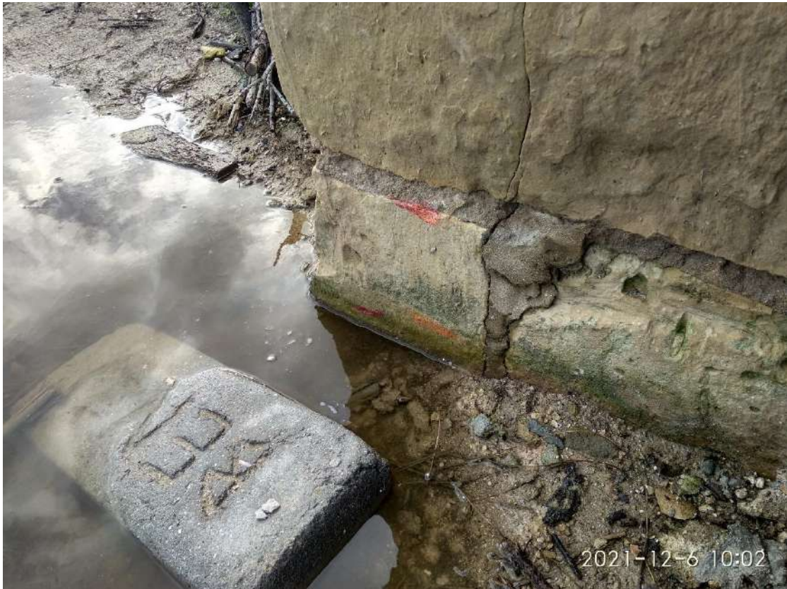
FIGURE 50: DECREASING WATER LEVEL AT NATURE TRUST TOOLS ROOM AS NOTED ON 6 TH DECEMBER, 2021
