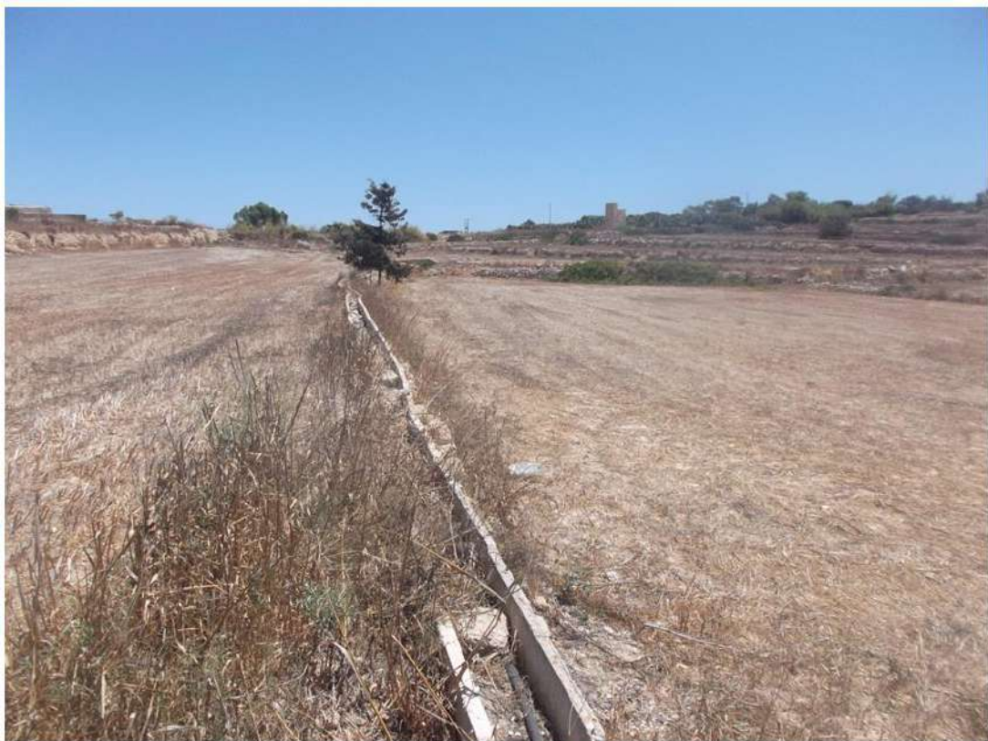
FIGURE 92: PHOTOGRAPH SHOWING THE IRRIGATION CHANNEL AT TAS-SILG. CHANNEL IS ABOUT 30CM WIDE
